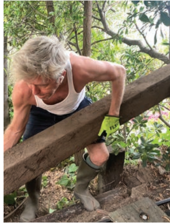
Removing timbers for retaining walls that were leaning and drifting downhill.
