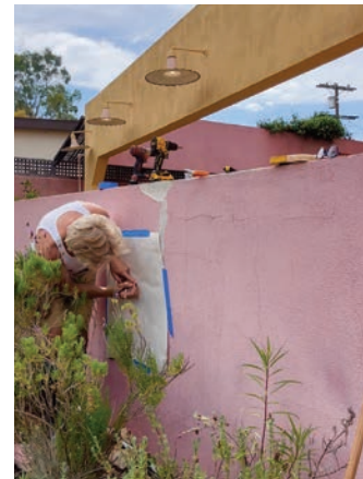
Cutting a paper template to patch a section of the courtyard wall.
