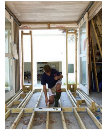
Building the diaphragms for the Dog Trot floor.
