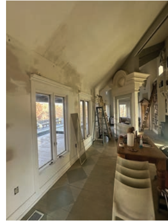
Water damage to the ceilings and walls was extensive.
