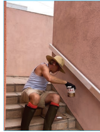
Priming newly restored railings.
