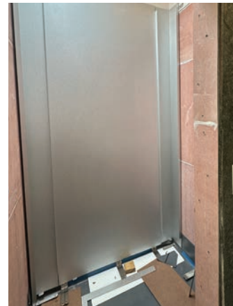
He also devised a new way to fabricate, hang, and seal the new steel panels for the shower walls.
