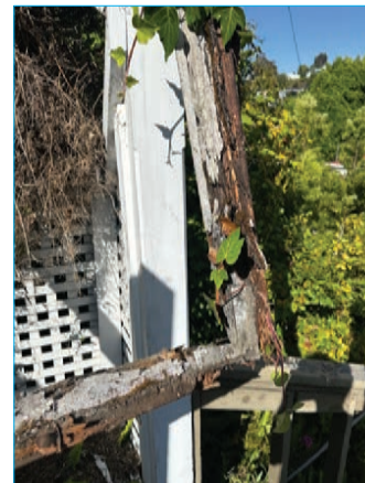
I had to demolish the all of the hillside railings and pergolas as they were rotting and in danger of structural failure.
