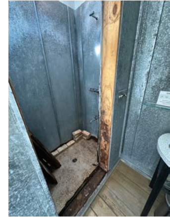
After removing the shower door, Kevin discovered the entire shower would need to be rebuilt because of significant rot and rust.
