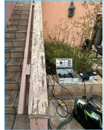
Sanding and scraping all of the staircase parapet caps.
