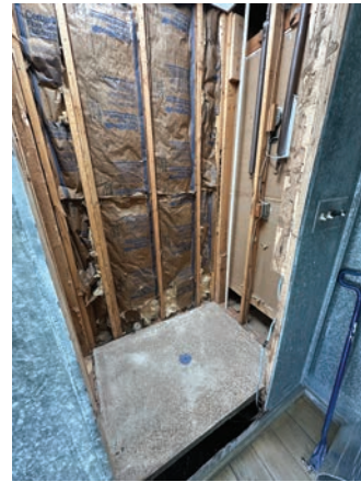
With tremendous effort, the old concrete floor had to be removed. Kevin rebuilt the entire floor, wall, and curb structure, whose members were rotting.
