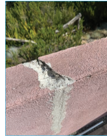
I am gradually repairing cracks, fissures, and pocks in the stucco.
