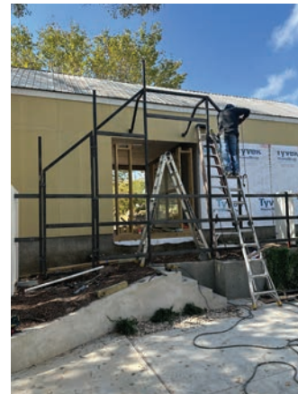
The metal fabricators welding the steel frame for the Western "false front".
