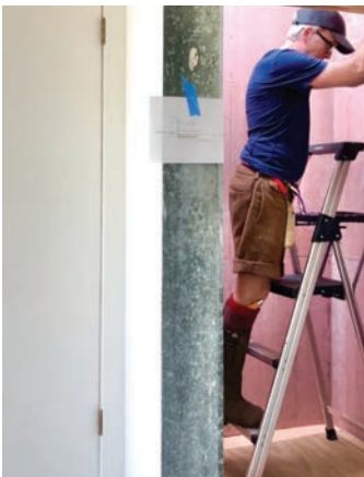
Hanging new water-resistant wall boards in the shower.
