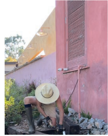
Pounding in re-bar to strengthen landscape retaining walls.
