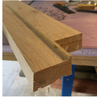
Shaping the new oak sill.
