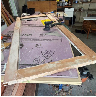
Sanding off layers of paint.
