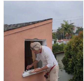
Caulking the glass perimeter.
