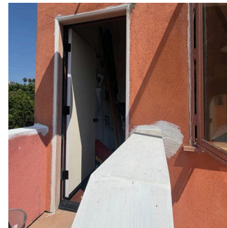
Installing new door moulding.
