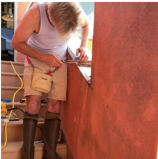
Removal of wall cap.
