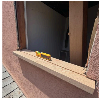
Installing the sill.
