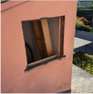
Removal of the entire window.
