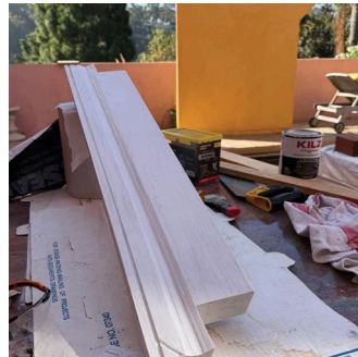
Oil priming the parts.
