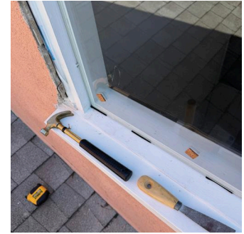
Mounting the new glass.
