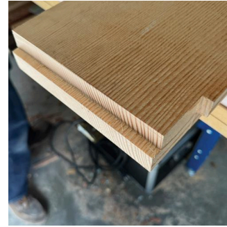
Planing and shaping the new rail.
