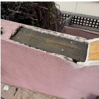
Repaired framing.
