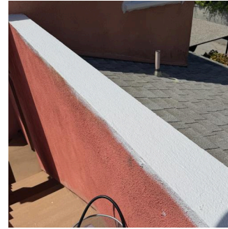
Sealing a wall cap.
